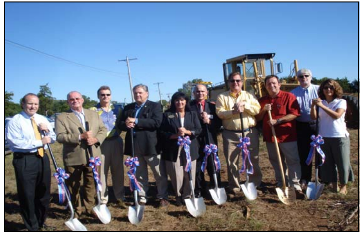
The ground was broken to begin construction for the new Fox Run Housing Development by the developer, chamber officials, PCDA officials and city leaders last week. This is exciting news for Ponca City! A great crowd was on hand for the groundbreaking event.
